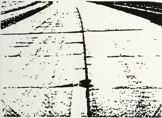
Fig. 3.2.3.7 — Joint separation
